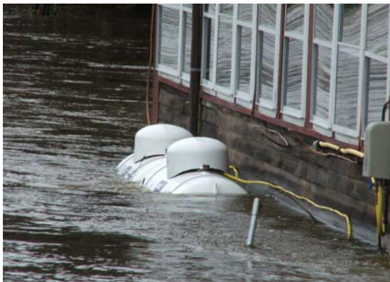
Hallowell April 2005, LP tanks not anchored and susceptible to flow. Photo by Bonnie Cowle, Maine Floodplain Management Program
