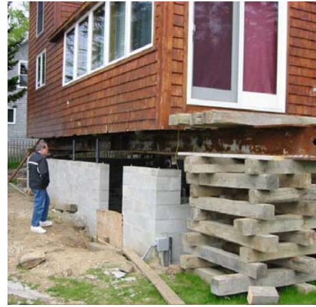
(Brunswick, ME) This structure is in the process of being elevated. Photo- Maine Floodplain Management Program
