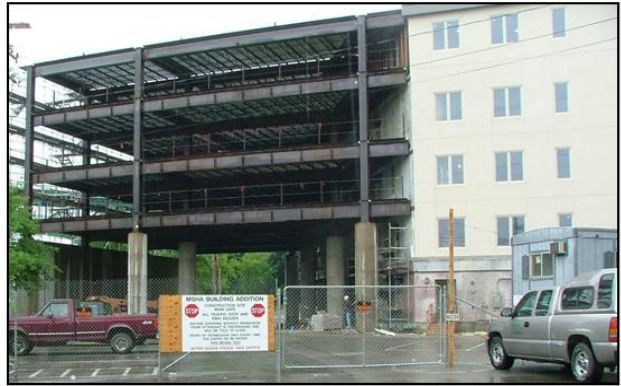
Augusta, ME. An addition to a commercial structure in the floodplain was considered substantial improvement. Flood proofing the older section of the building included retrofitting with a rubber lining. Photo Lou Sidell, Maine Floodplain Management Program
