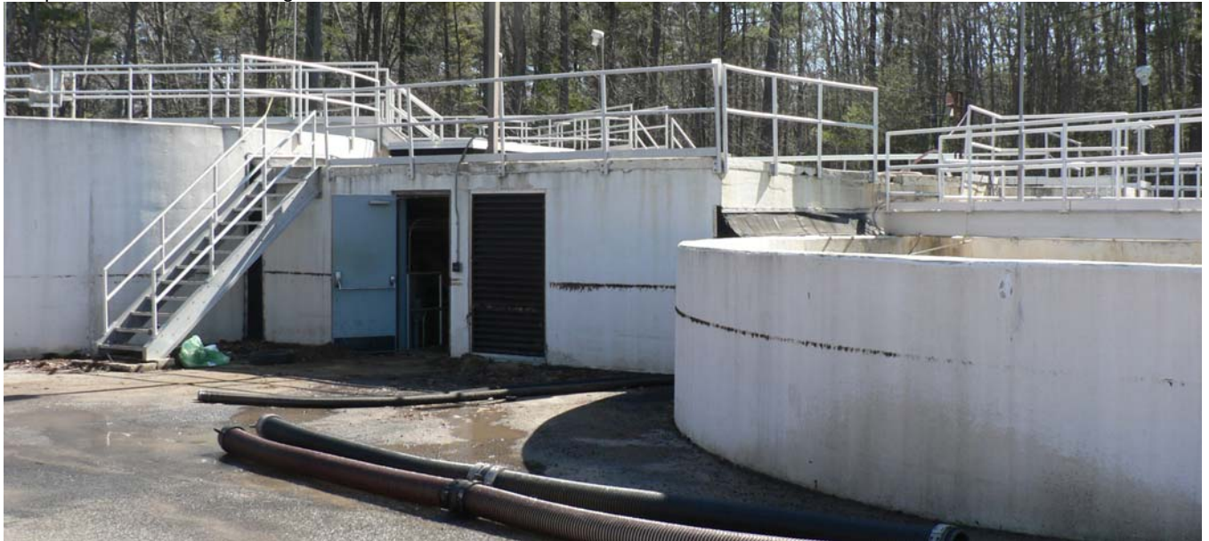
(Kennebunk, ME) Critical facilities located in the floodplain are at risk. Photo by Lance Carpenter, FEMA.
