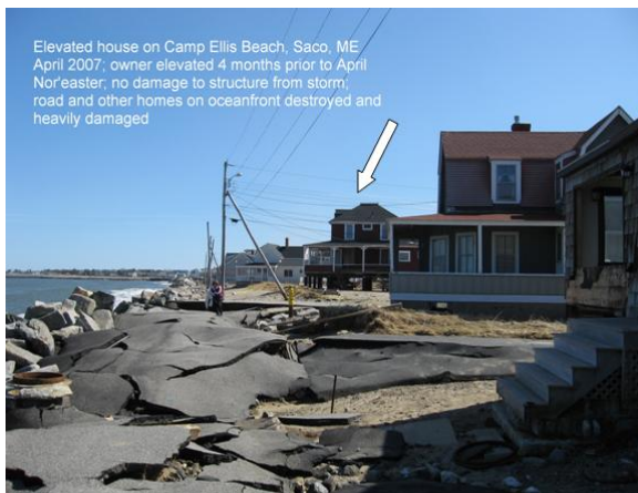
(Saco, ME) Property owners who elevated home four months prior to April 2007 nor'easter did not sustain damages as a result of that storm. Photo courtesy of Town of Saco Emergency Management.
