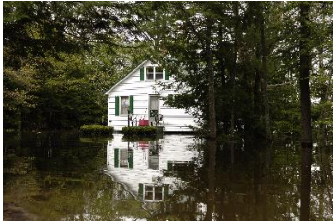
(Shapleigh, ME) Houses located near rivers and lakes in York County were surrounded by high water for many days after heavy rains inundated the region in May, 2006. Photo by Jocelyn Augustin.
