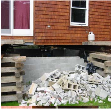
(Brunswick, ME) This structure is in the process of being elevated. Photo- Maine Floodplain Management Program
