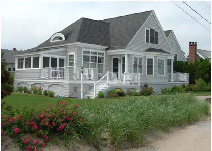
(Saco, ME) Mitigation measures such as bolting vertical surfaces to the foundation and using hurricane-resistant shingles paid off for owners of this home during 2007 Nor-Easter.
