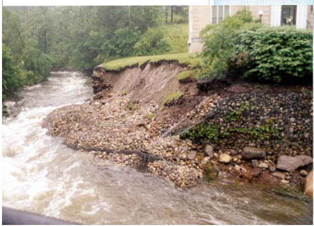
(Wilton, ME) (Left) Floods in 1999 caused gabion wall outside of the Wilton Free Library to collapse. (Right) This concrete wall was erected to protect the Wilton Free Public Library in 1999 and has held up through many floods. Photos courtesy of the Town of Wilton.
