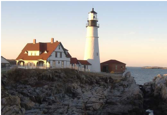
(Cape Elizabeth, ME) The Portland Headlight is an example of a historic structure located in a floodplain. The light, housed in one of New England's handsome cast-iron lighthouses, still acts as a navigational aid. The U.S. Coast Guard maintains its equipment.
