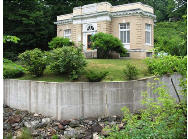
(Wilton, ME) (Left) Floods in 1999 caused gabion wall outside of the Wilton Free Library to collapse. (Right) This concrete wall was erected to protect the Wilton Free Public Library in 1999 and has held up through many floods. Photos courtesy of the Town of Wilton.
