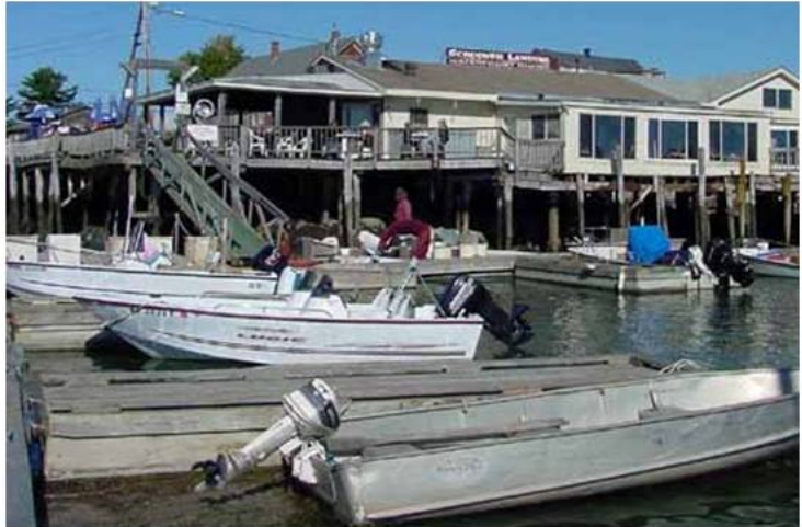
(Damariscotta, ME) Schooner Landing – when this property was sold the insurance and insurance rate was transferred to new owner (grandfathered). The structure would be uninsurable under current NFIP standards. Photo by Bonnie Cowle, Maine Floodplain Management Program.
