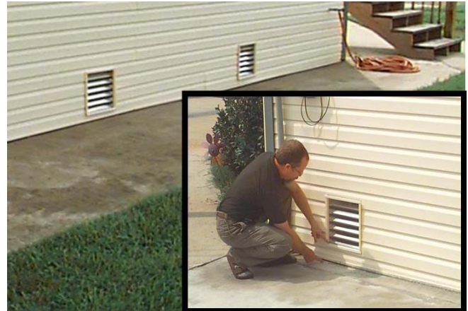
A code inspector measures height of flood vents which allow floodwater to flow underneath a building.
