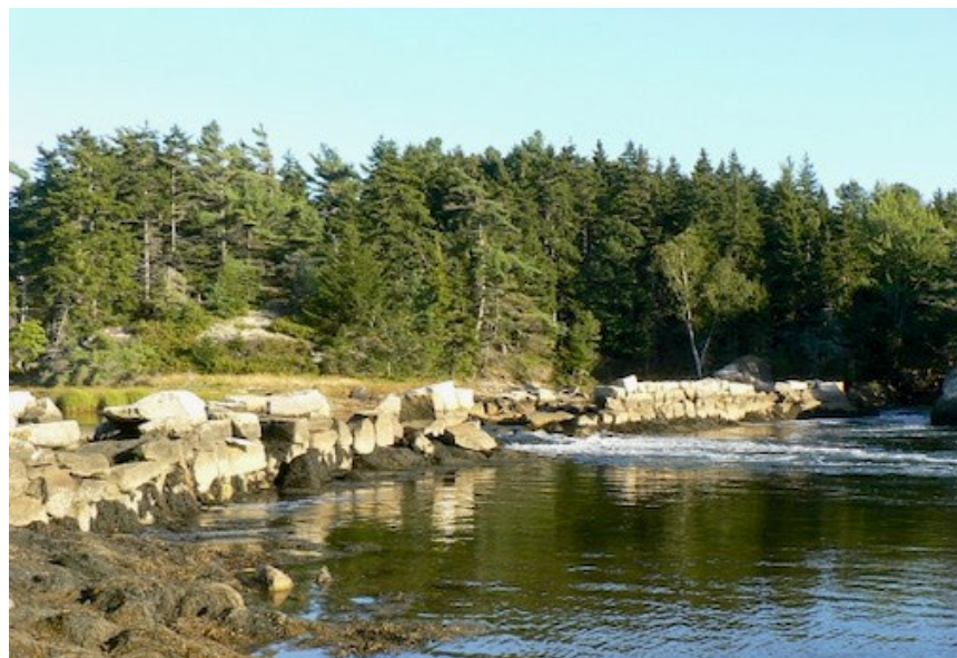
Image 1. Dam at the western side of Spirit Pond. 6
