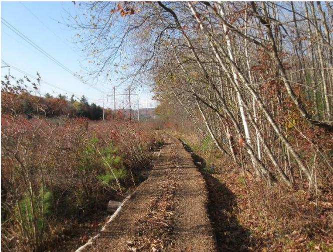
Begin your turnpike by clearing the site wide enough for the trail tread plus a ditch and retainer log or rocks on either side of the trail tread. Rocks, stumps, and stubs that would protrude above the turnpike tread or cause rips in geotextile fabric should be removed or at least cut flush below the final base grade.
