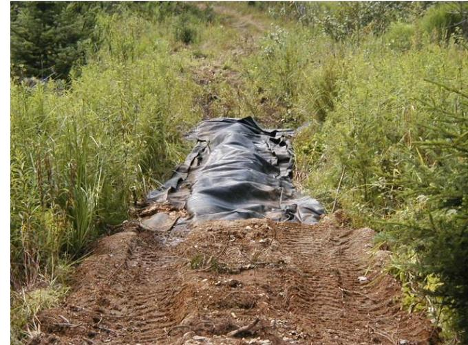
**Geotextiles**, commonly called construction fabrics, are often used in trail turnpike construction. They are made from long-lasting synthetic fibers bonded to form a fabric. They serve as a barrier between the mucky saturated soil beneath the fabric and the mineral or granular soil placed on top.
