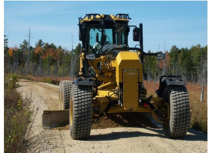
Regular grading or raking is an effective means of redistributing material that has either been washed or pushed to the edge by vehicle traffic. Over time, as the soil compacts, a berm will often form at the downhill edge of the trail. These little ridges defeat the purpose of crowning by preventing water from draining off.
