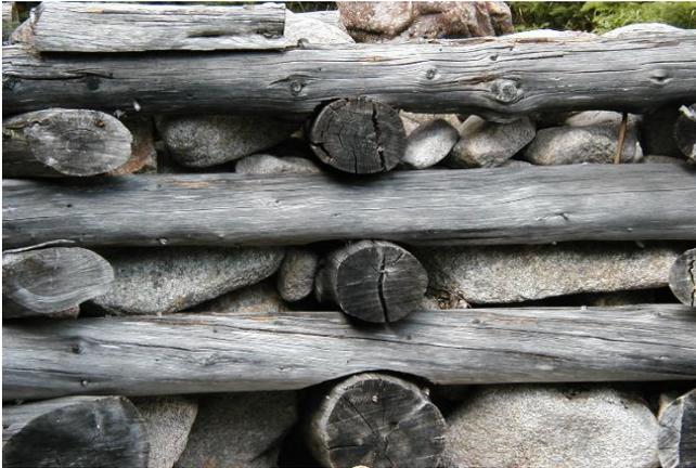
Construct a wood crib by interlocking logs or beams and pinning them at the joints. Be sure to select Pressure treated or peeled rot-resistant logs such as Hemlock or Cedar. Lay sill logs at right angles to the direction of travel and alternate tiers of face logs and header logs. Add rocks to plug the space between the logs.
