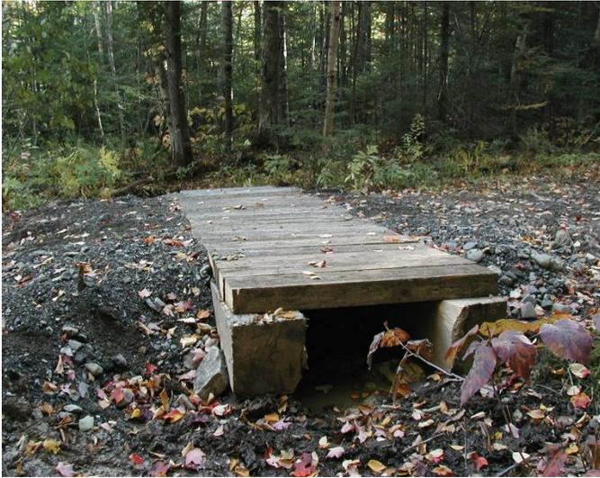
**Wood Box culvert: no gravel cover needed**
